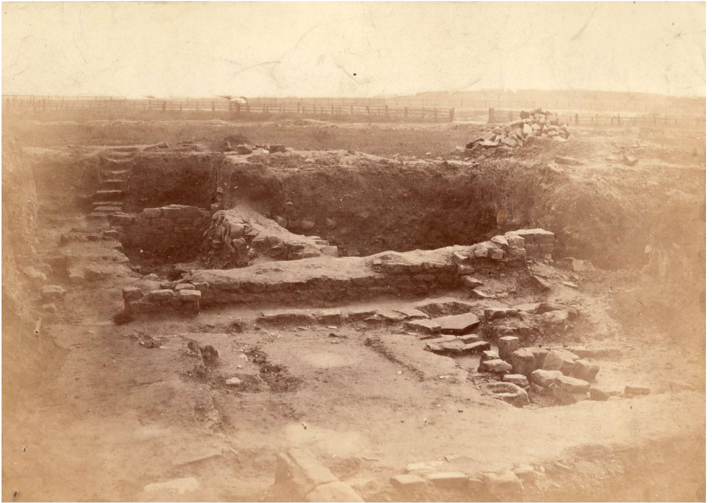
Fig. 55: The hypocaust in building X (front right), looking south. There is a socket stone in its near corner. The wall running across the centre with the remains of two buttresses is the north wall of granary C16. Note the wide open fields of Field House Farm (the Shieldsheugh estate) beyond the fence.
