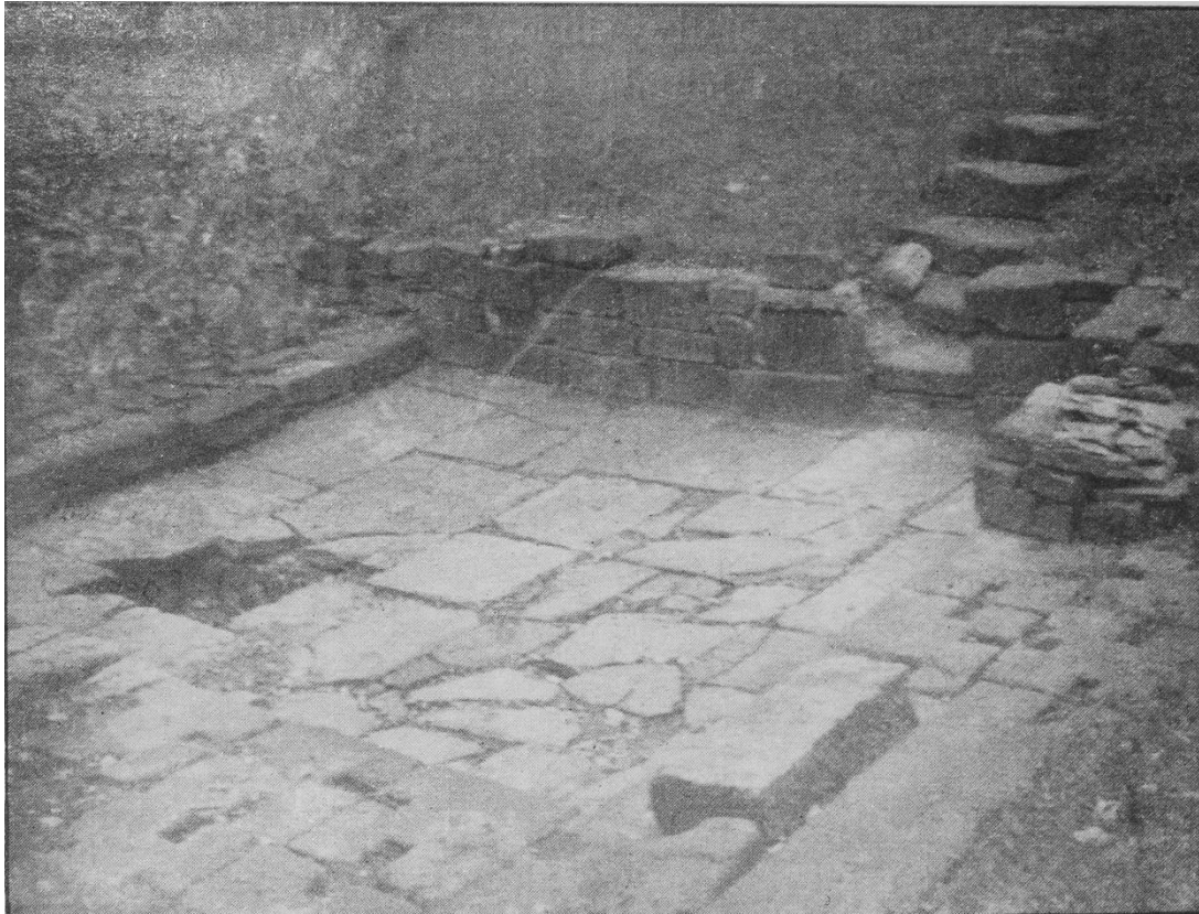
Fig. 66: The strong-room of the headquarters building, taken from Hodgson 1903, so probably similar in date to Fig. 65. The window stone with holes from iron bars is visible perched on the low wall at the back (cf Fig. 65), but the jamb and the lower window stones (see Figs 47-8) have vanished. To the right stones have been removed from the west wall to reveal two lines of the big blocks with clamp sockets; originally there were large blocks on top of the outer row (cf Fig. 47).
