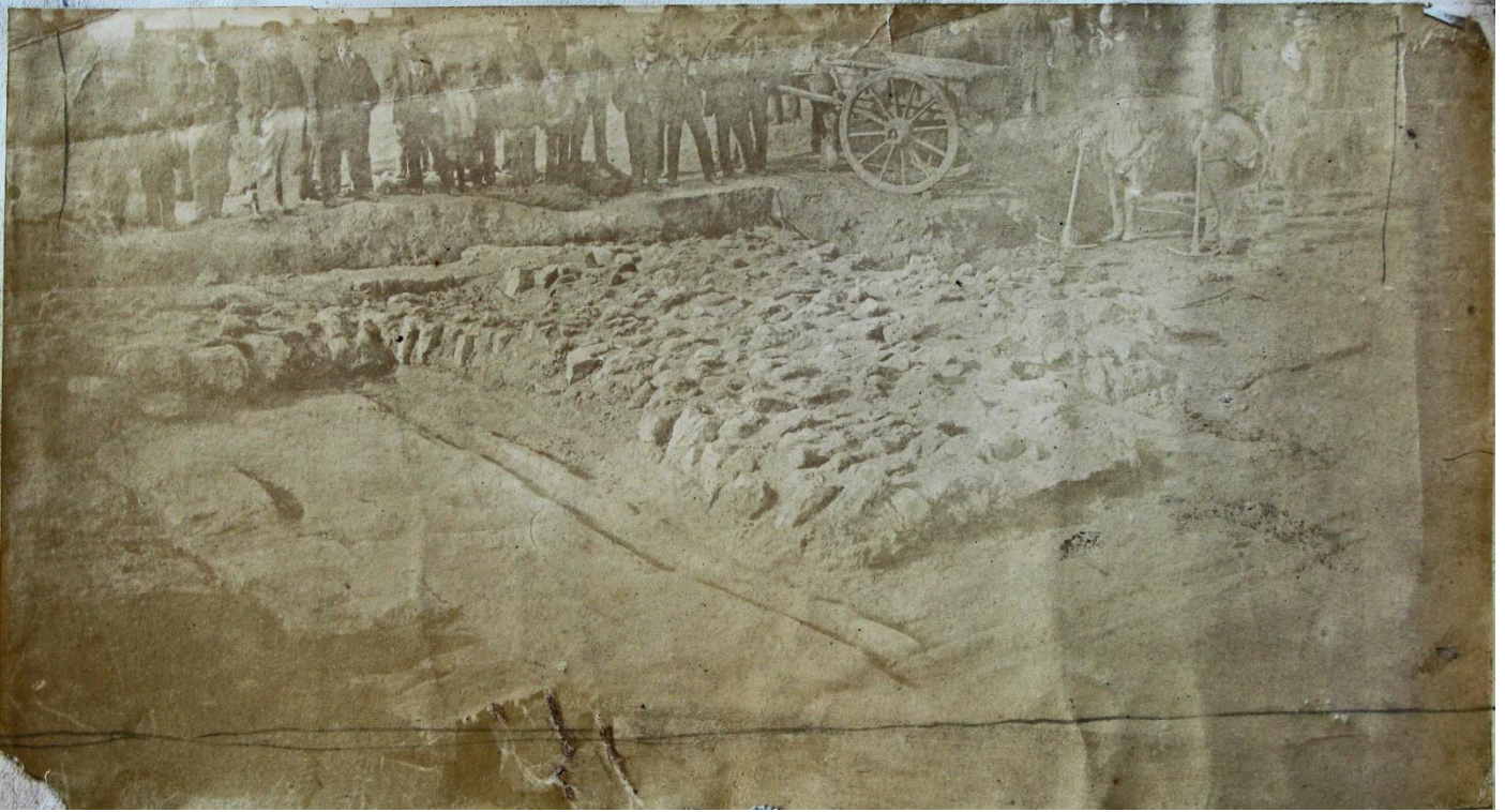
Fig. 43a: Forecourt of the headquarters building with the fallen wall, looking north-east. This photo was taken at a later date than Figs 41-2 since the individual stones of the fallen wall are now visible.
