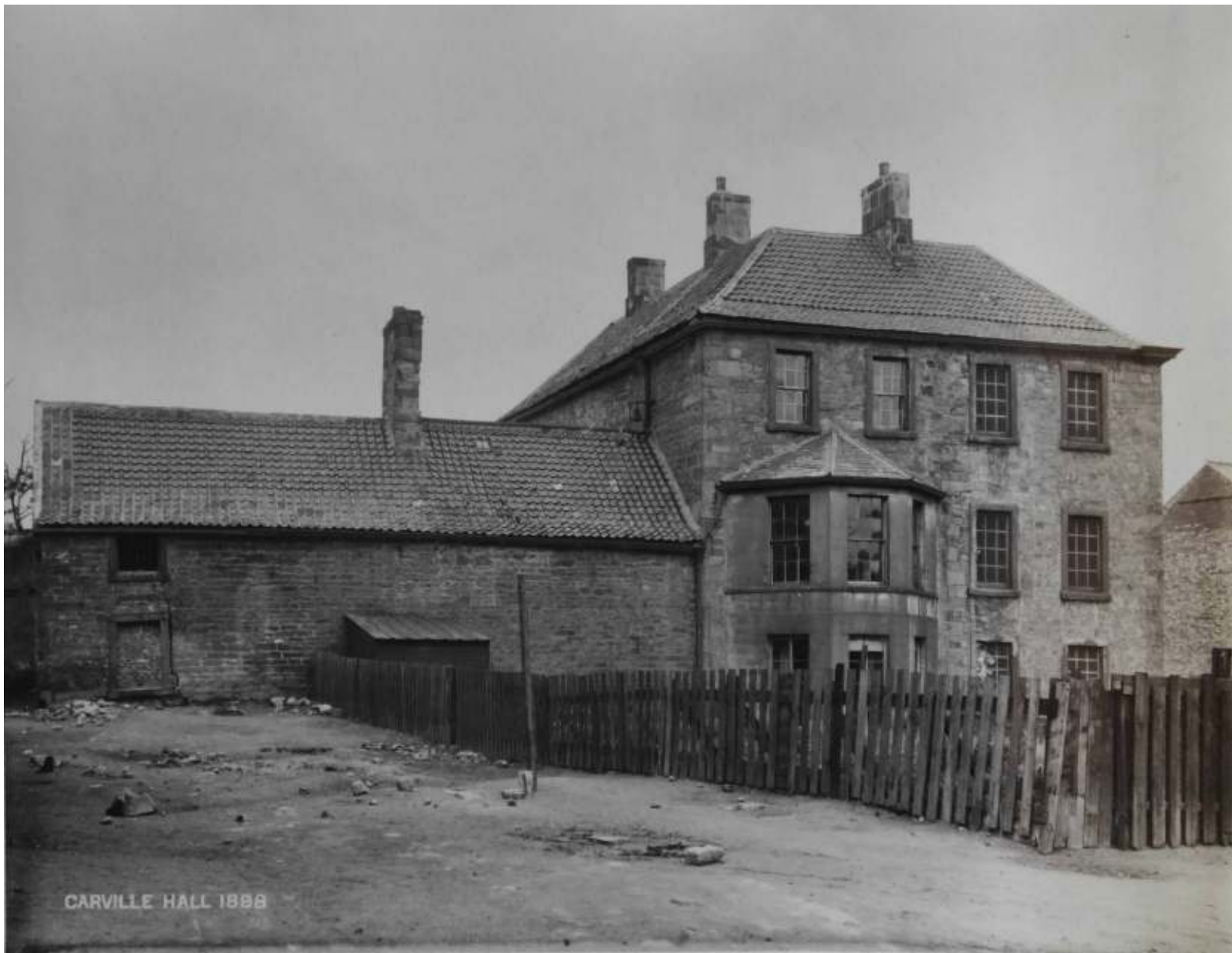
Fig. 13. Carville Hall in 1898, from the west, showing the service wing. Note the two columns of blocked windows on the right-hand side. This side of the house has four windows across, while there are only three on the east side (TWAM DS.SWH/4/PH/6/2).
