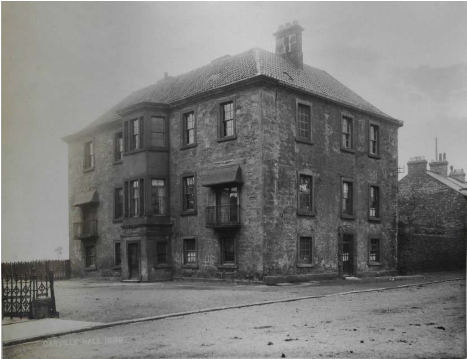
Fig. 12. The front and east side of Carville Hall in 1898. The three windows on the left-hand side of the east face have been blocked in and painted (TWAM DS.SWH/4/PH/6/2).
